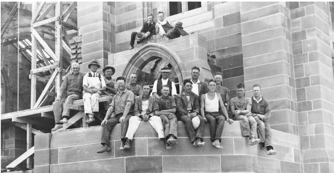
Construction workers at St Andrew's circa 1932/33
